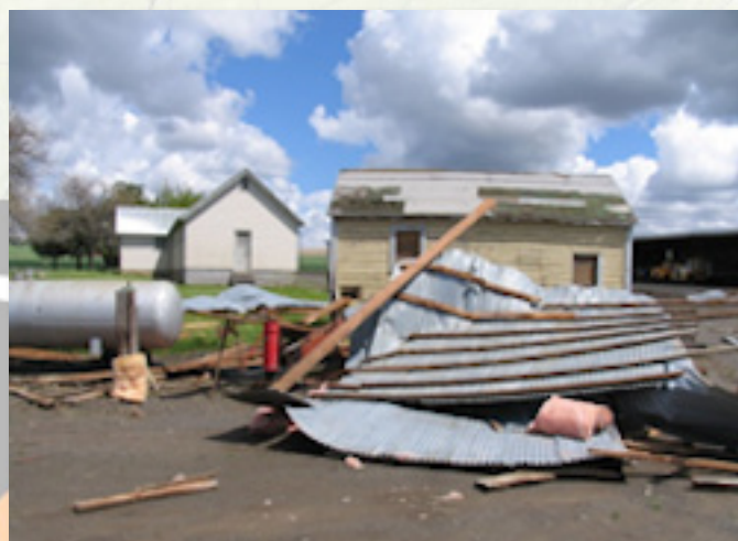
Tornado damage southeast of Adams OR, May 2009
