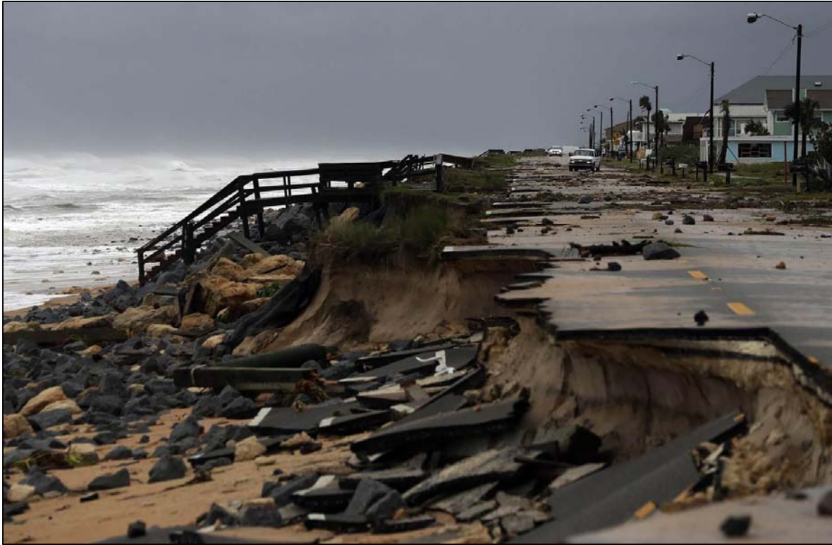
Figure 12: Beach erosion and road damage on Highway A1A left by Hurricane Matthew in Flagler Beach, FL. Source: NBC News
