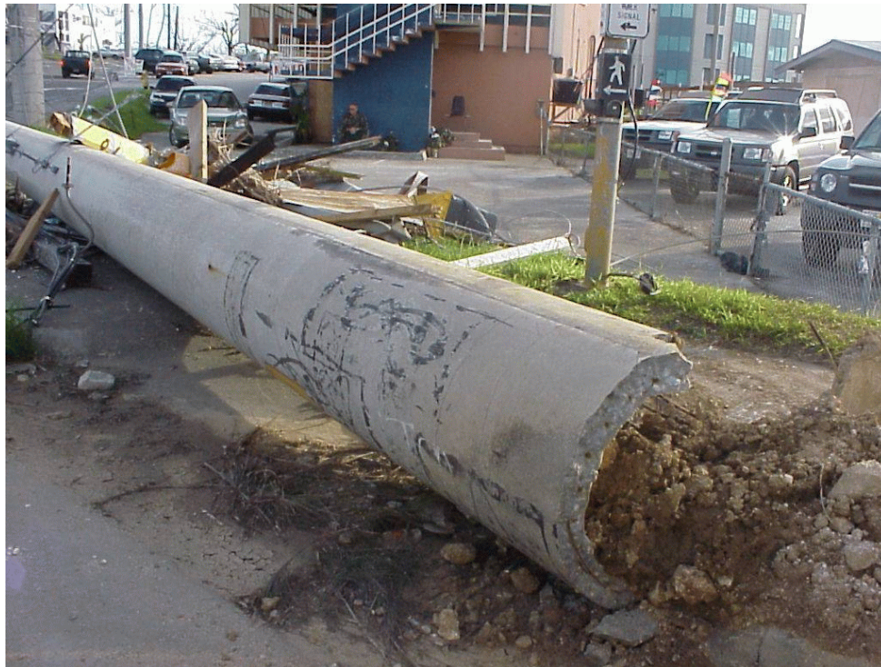
Downed utility pole along a back road east of the Bank of Guam (upper right) in Agana, Guam. (NOAA)
