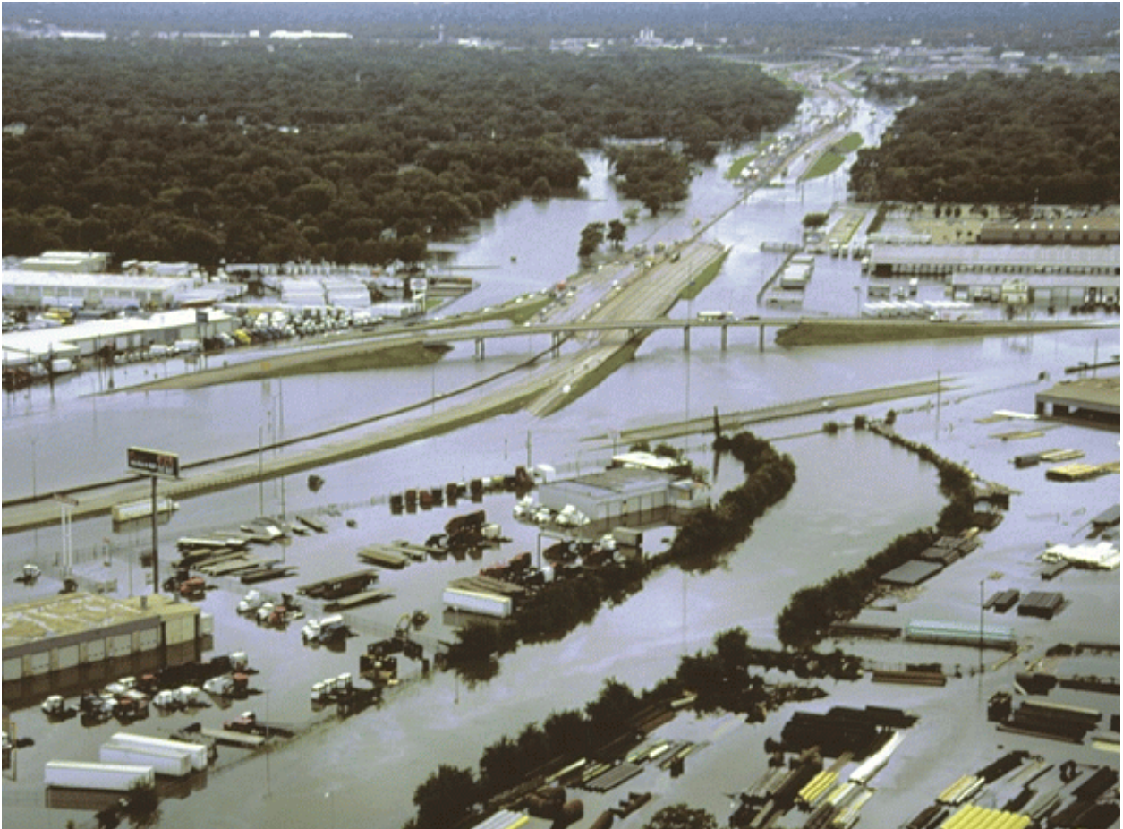
Interstate 10 North Loop, Houston, Texas. (Courtesy of Harris County Flood Control District/ Steve Fitzgerald)
