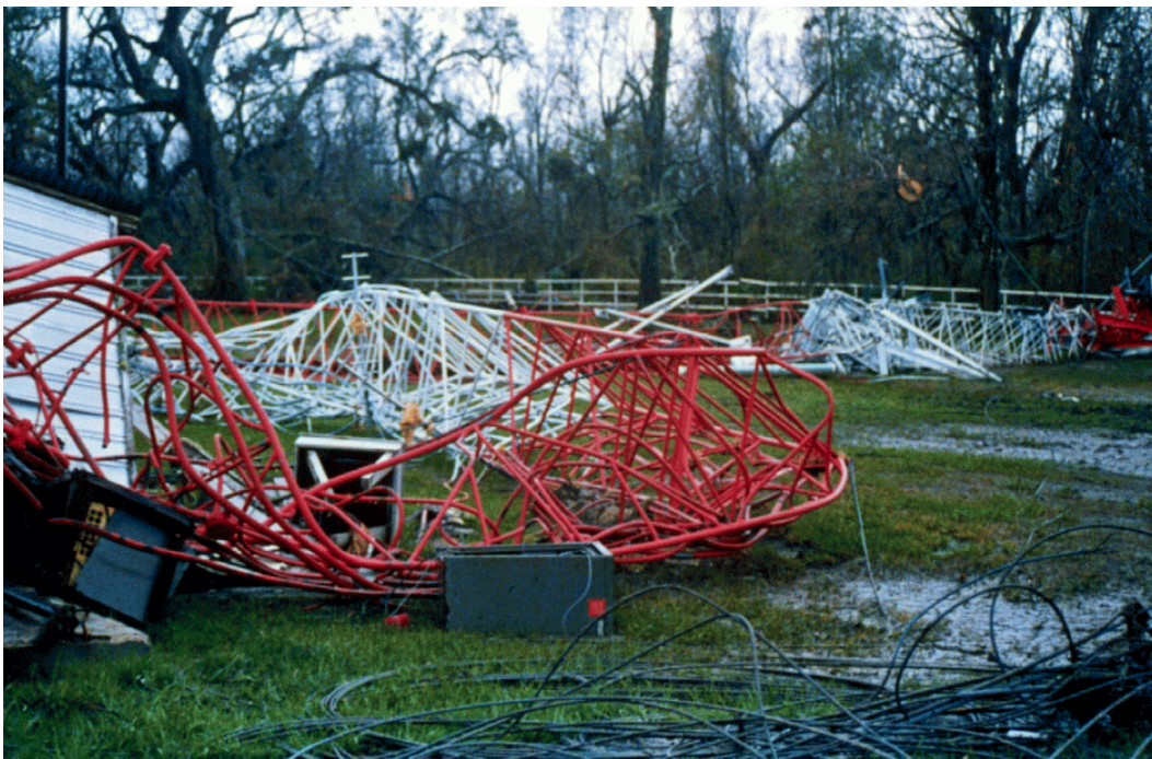
Tangled remnants of what was once a radio tower along U.S. 90, south of Centreville, Louisiana.
