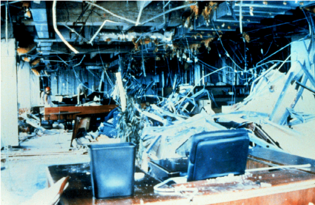
This photo depicts wind damage to the top floor of the Burger King World Headquarters building.
