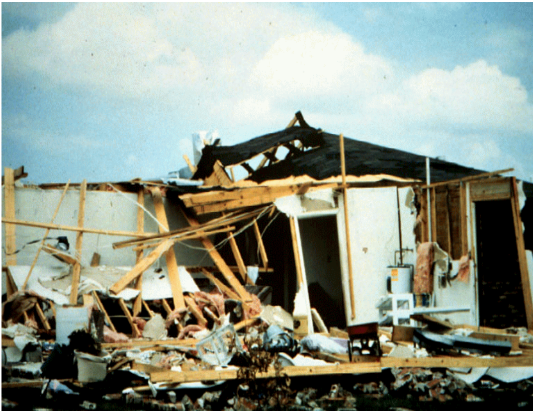
F-3 tornado damage to the communities of La Place/Reserve located 30 miles west of New Orleans, Louisiana.
