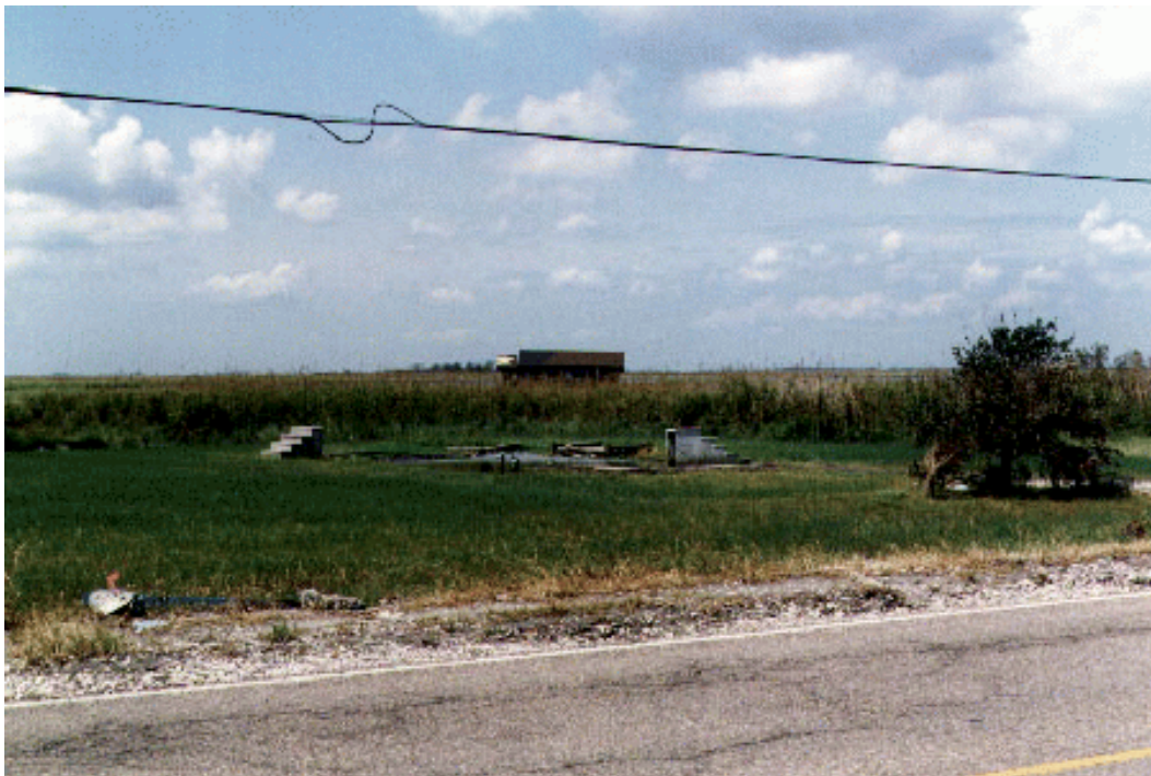
North of Cocodrie, Louisiana, home in the background was removed from its foundation by a combination of storm surge and wind.
