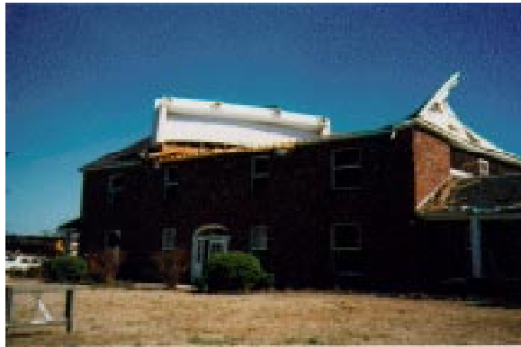
Photograph of brick church in Arkadelphia with major roof damage and broken windows. This church was on the edge of the downtown area where major destruction occurred. Courtesy of Chris Smith, NWS Southern Region.
