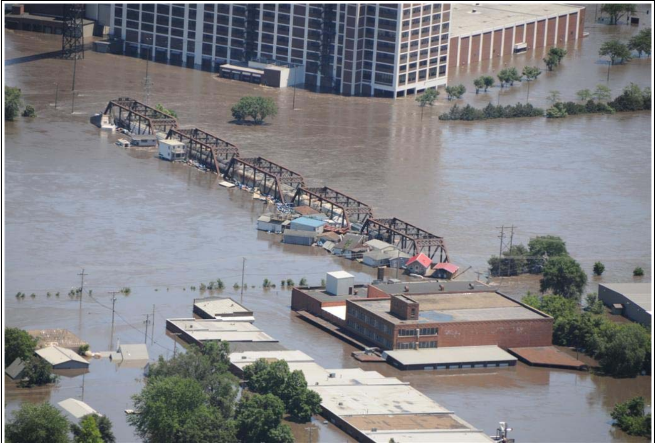
Fig. 30. Houseboats were carried by the Cedar River into the railroad bridge near the Quaker Oats plant in Cedar Rapids, Iowa. (Used with permission. ©2008 Iowa Homeland Security and Emergency Management Division. Photograph by the Civil Air Patrol.)
