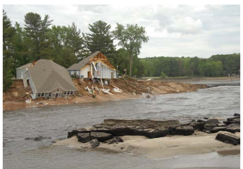
Fig. 14. Homes were destroyed on Lake Delton in Wisconsin when the 245-acre lake quickly emptied after Dell Creek cut a new channel into the Wisconsin River, bypassing the dam. (U.S. Air Force photograph by Master Sergeant Paul Gorman.)
