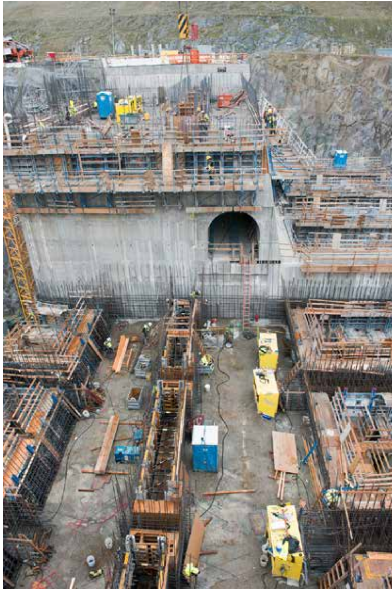
The Folsom Dam auxiliary spillway construction site on February 26, 2014. Photo Credit: Courtesy of California Department of Water Resources, Florence Low
