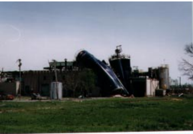
Damage to Industrial Buildings, Clayton Parkway, Ft. Smith
