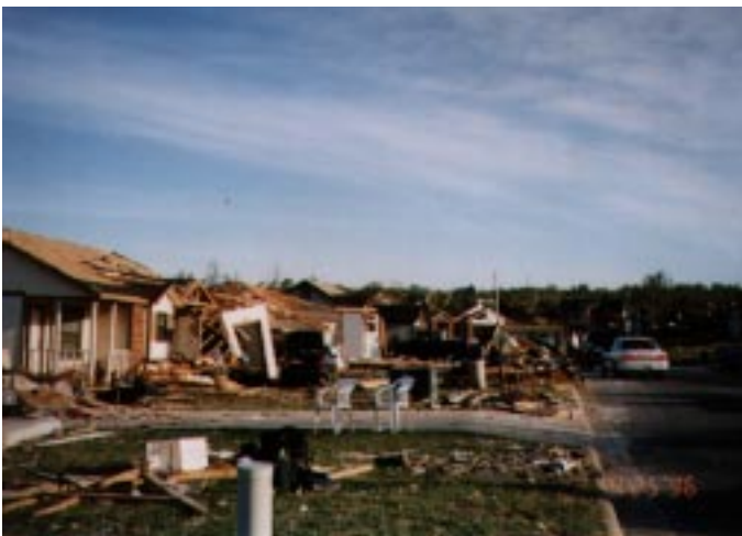
F3 Damage, Vista Ridge subdivision, Van Buren
