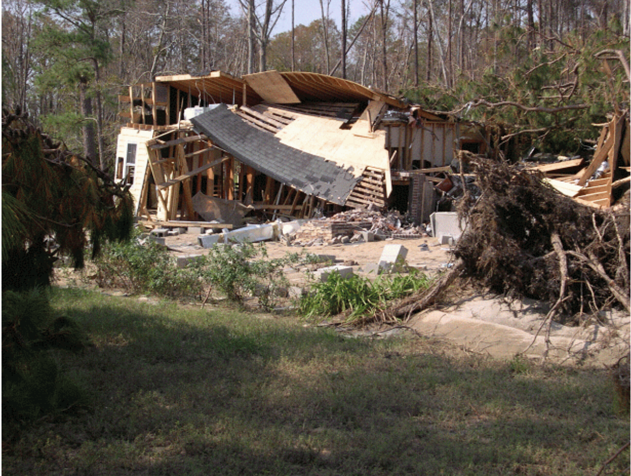
Picture 2. A small cluster of four homes about 5 miles west of Edenton, NC, occupied year-round were completely destroyed by the surge, two of which were moved up to 20 feet off their concrete block foundations. (NWS Isabel Assessment Team photo by Dave Vallee.)
