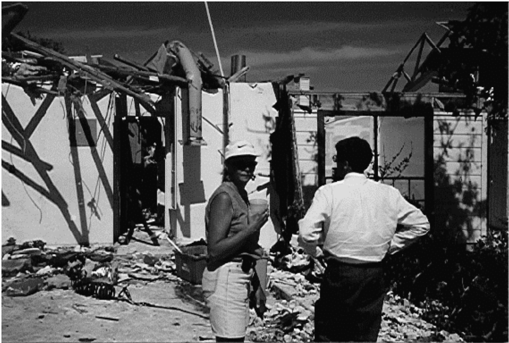
Home destroyed in Buttercup Creek subdivision during Cedar Park tornado. Several people took shelter in a utility closet, shown just to the left of the woman in the picture. Photograph by NWSFO Austin/San Antonio.
