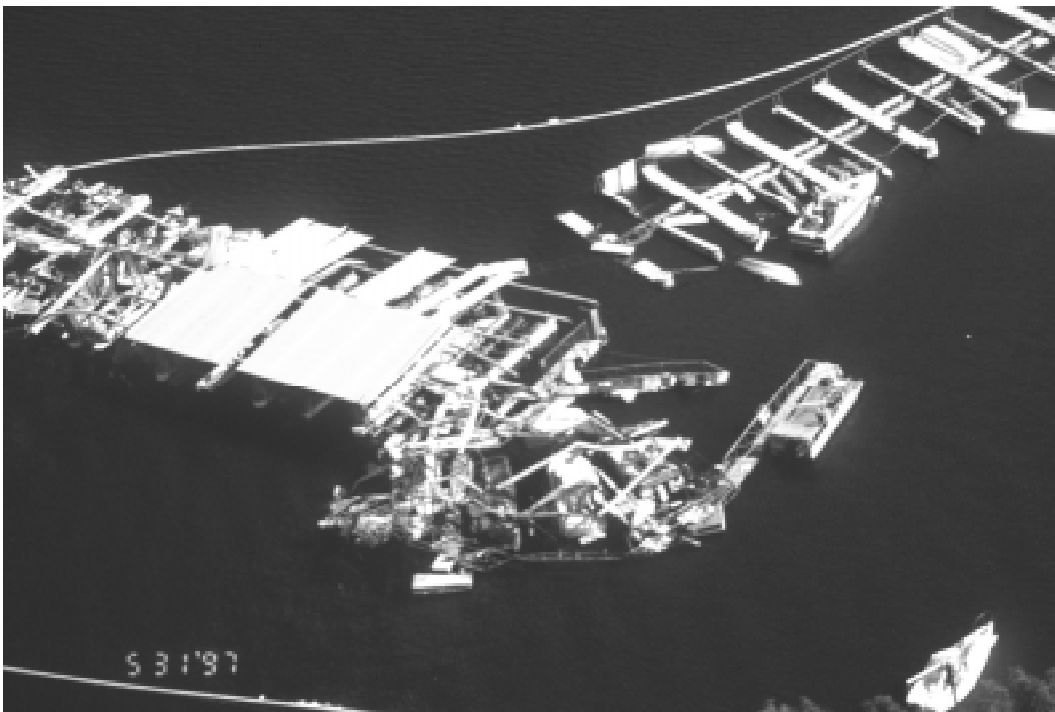
Aerial view of damage to boats at Belton Lake from the Belton tornado. Photograph by L. Phan, NIST.
