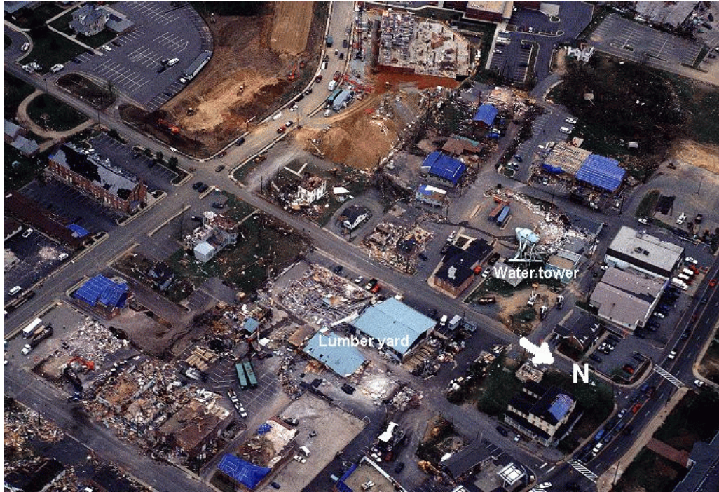
Photo 3. Aerial view of a lumber yard and downed water tower in downtown La Plata, Maryland. (Courtesy of Tim Marshall, Haag Engineering)
