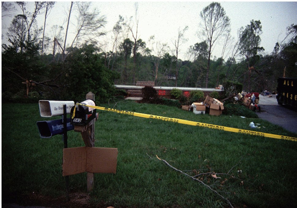
Photo 6. Poorly anchored home on Morgans Ridge Road was swept clean off its foundation while mailboxes remained undamaged. This example illustrates the difficulties in assigning an F-scale rating. (Courtesy of Tim Marshall, Haag Engineering)
