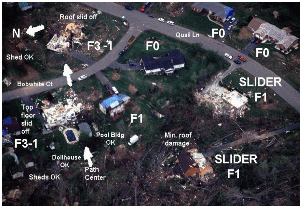
Photo 4. Aerial view of residential damage in the Quailwood Subdivision looking east. Several poorly attached homes slid off their foundations and rated F1. (Courtesy of Tim Marshall, Haag Engineering)
