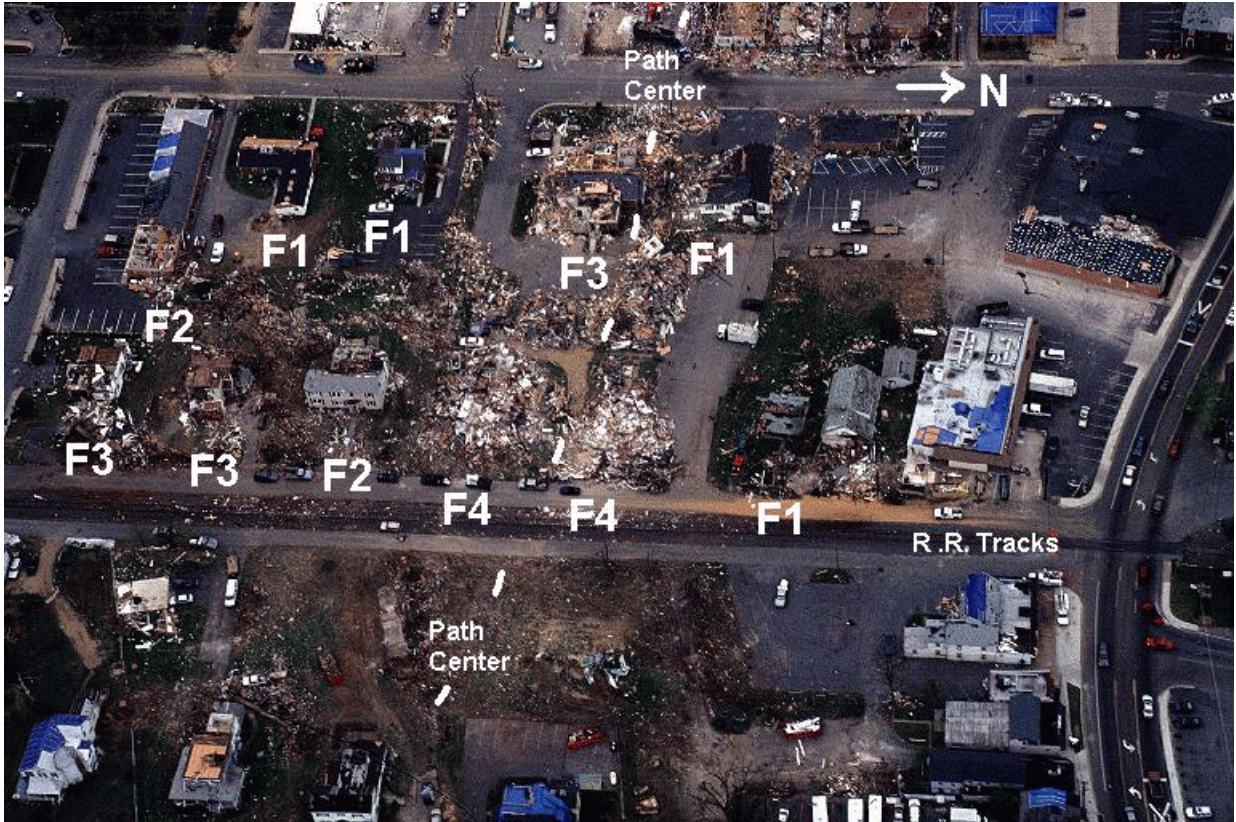
Photo 2. Aerial view showing F4 damage to two homes in downtown La Plata, Maryland. These homes were downwind of a lumber yard and impacted by its debris. (Courtesy of Tim Marshall, Haag Engineering)
