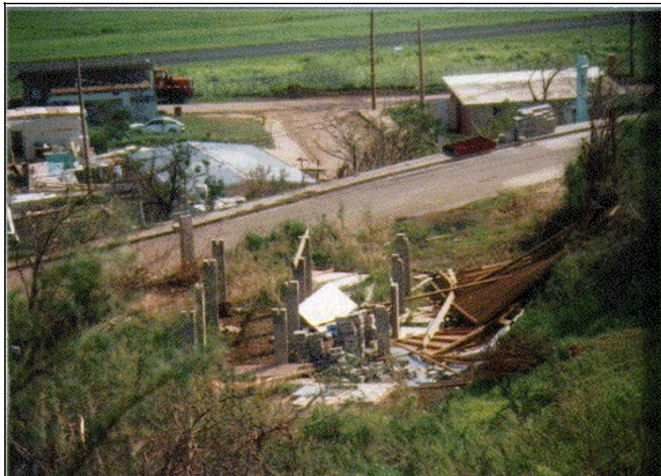
Figure 1-19. Home flipped off its pilings. (Photo courtesy of Reggina Garza)
