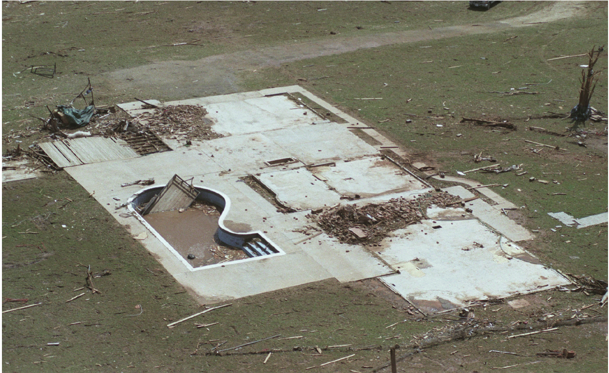
F5 damage to a home in Moore, Cleveland County, Oklahoma, May 3, 1999. Note most debris has been blown away. (Photograph copyright 1999. The Oklahoma Publishing Co.)
