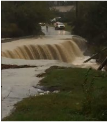
Road washed out on Greenock Avenue in Fayetteville. Photo taken by Fayetteville Police via WNCN.
