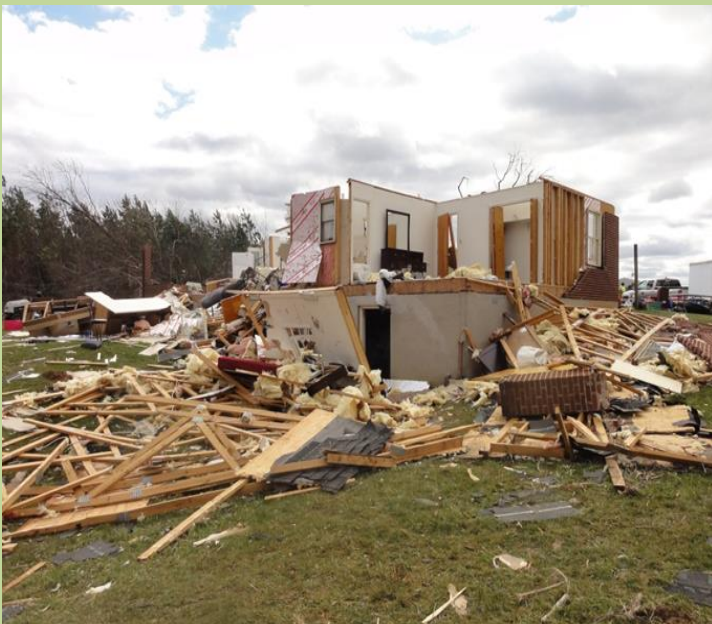
Damage to a home in the Evergreen area
