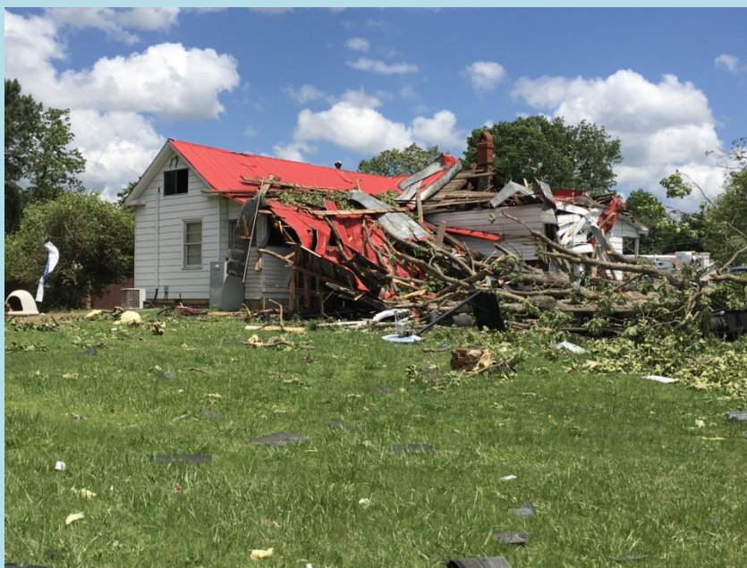
Damage from EF1 tornado in Eden, NC – May 5, 2017
