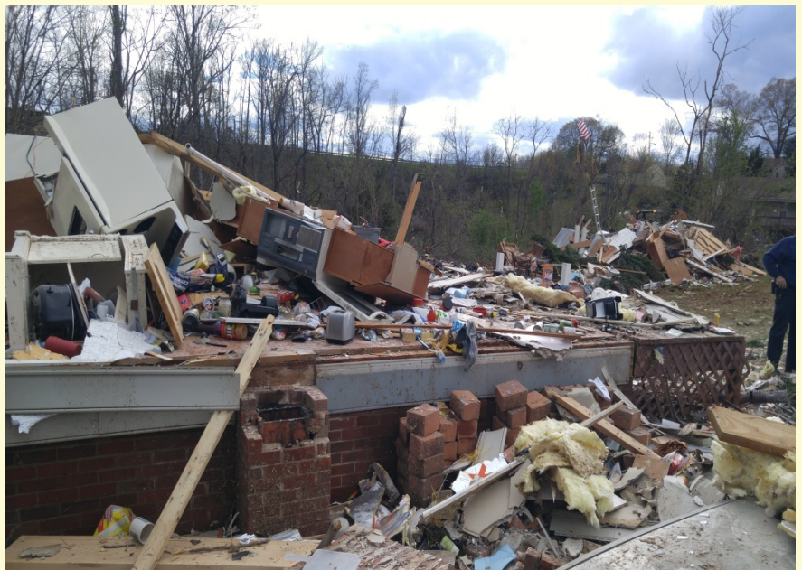
EF3 tornado damage in Elon, VA - Apr 15, 2018
