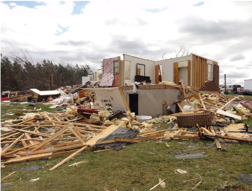
Fig. 7a. Damage to a home just south of Evergreen, VA near the start of the tornado track.
