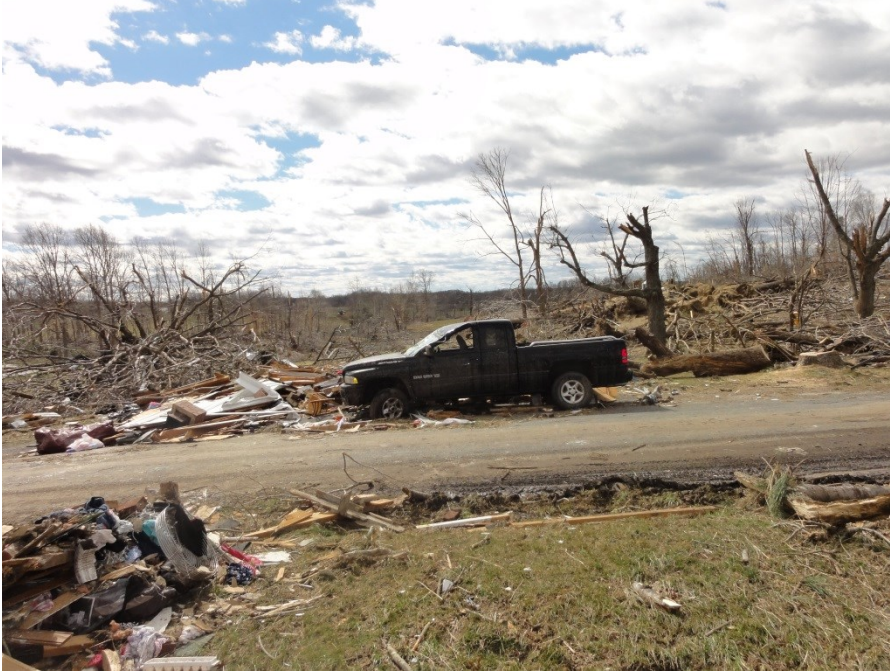
Fig. 7d. Damage to structures and trees, as well as a truck in Evergreen.
