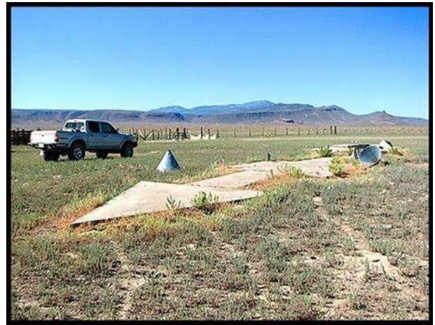
Figure 1 – Giant concrete navigation arrow.
